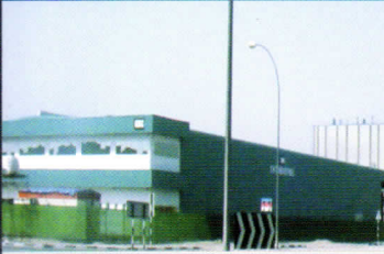
PLANT I, DUBAI
