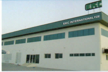
PLANT II, DUBAI
